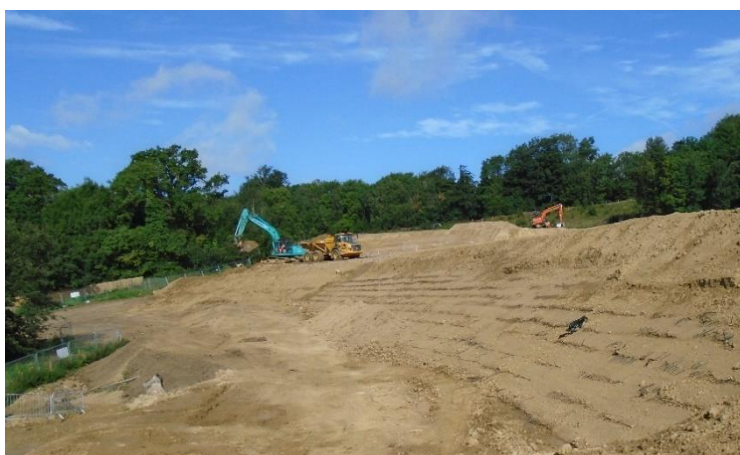
Figure 5. Shallow slope during construction at the Queenway Gateway Link project where the drainage geogrids are placed in layers at equidistance vertical centers; the facing element of the slope will be created using hydro seeding over an erosion geosynthetic mat.
