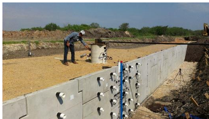
Figure 30. Construction of the MSE wall.
