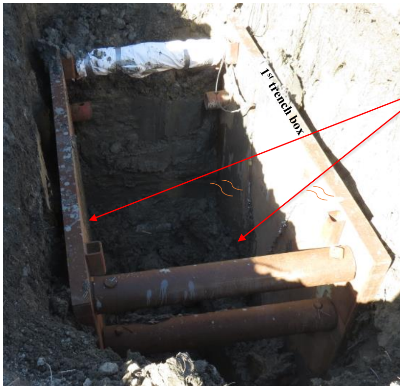
Figure 23. Likely “fixed end condition” developed at the lower end of the first trench box due to 300 mm insertion into the soil.
