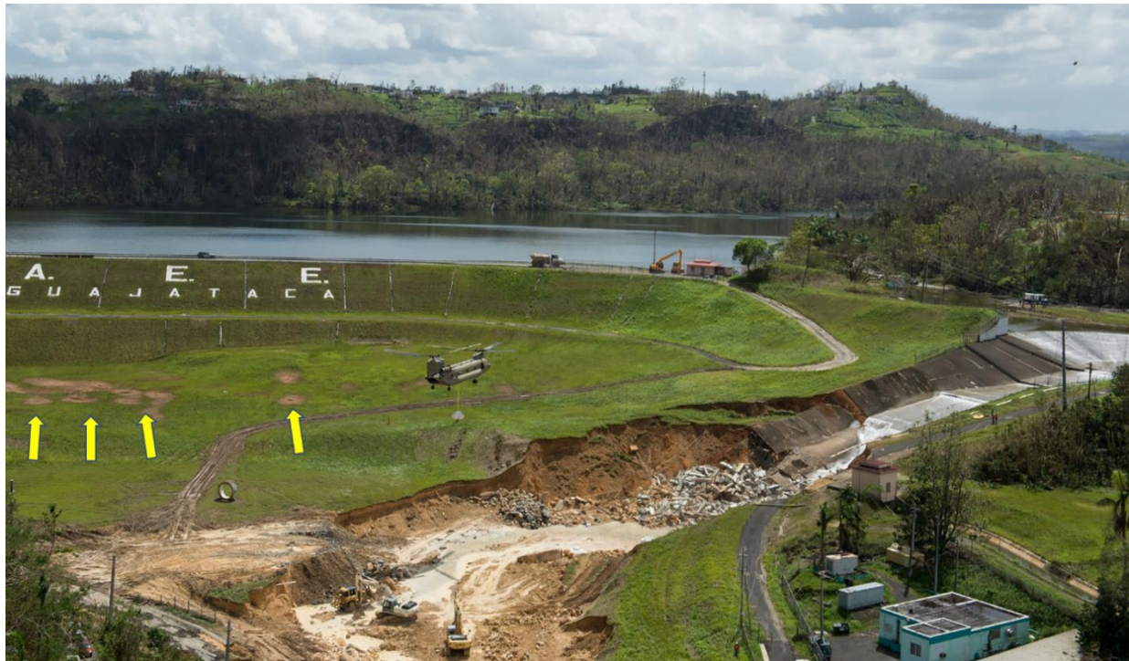
Figure 12. Apparent sand boils downstream of the dam toe (photograph from the Pennsylvania National Guard; figure adapted from Silva-Tulla et al., 2018).
