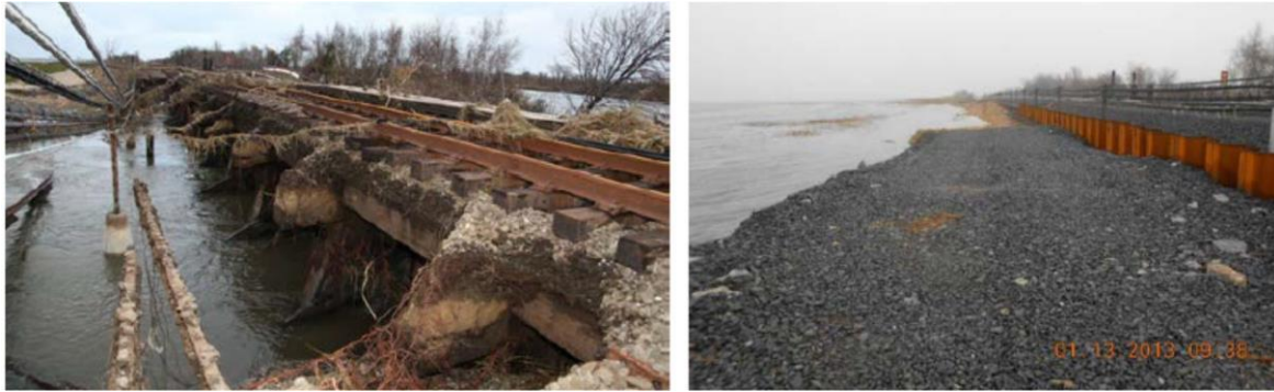
Figure 16. Earth embankment washouts in Queens, along Rockaway subway [A] line after Sandy with old LIRR infrastructure exposed (left) and post mitigation work (right). Photos by Khinda, ed. (2013).
