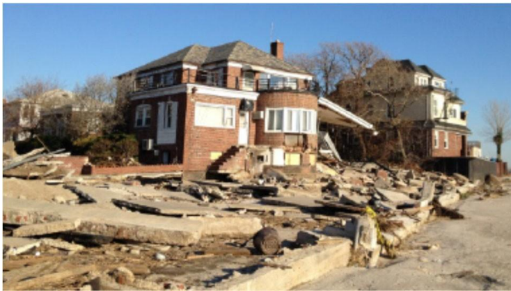
Figure 20. Undermining of beachfront retaining wall and loss of retained soil, Sea Gate, Brooklyn (left, 11/9/12); Destroyed CMU wall foundation, Breezy Point, Queens (right, 11/12/12). Photos by NYCDob (GEER, 2014).
