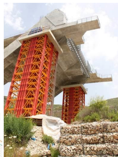
Figure 10. Arrangement of the MT towers beneath the curved struts of the bridge pier.
