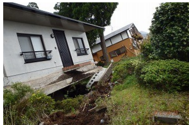
Figure 33. Damage to the house in residential area developed by filling (Site 21 in Fig. 26) ( 32^{\circ} 52'45.06''N , 131^{\circ} 00'1.44''E ).
