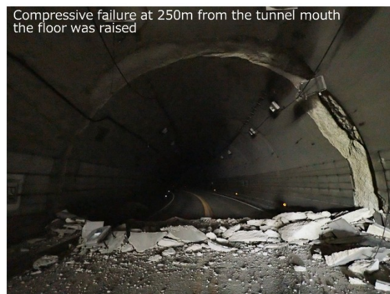
Figure 25. Tawarayama tunnel suffered from axial compression failure (Site 16 in Fig. 12) ( 32^{\circ} 51'35.68''N , 130^{\circ} 58'6.86''E ).
