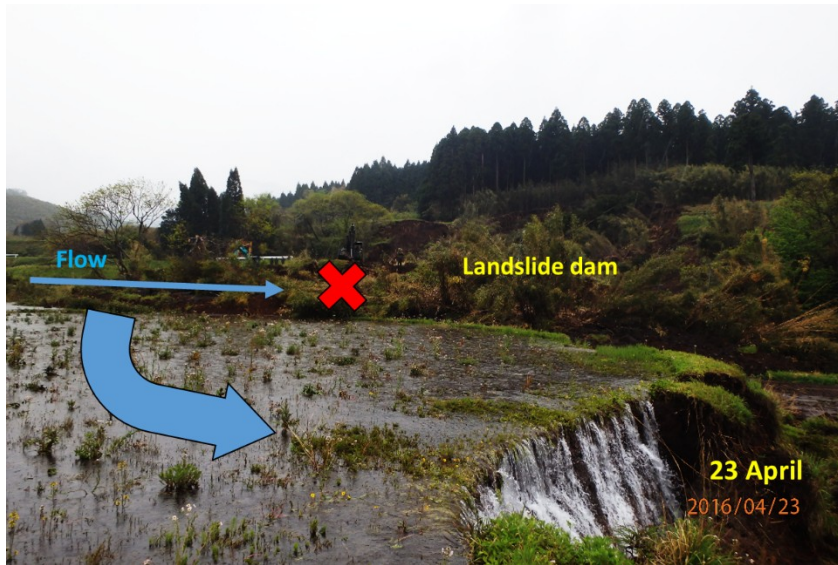
Figure 31. Landslide dam formed by the earthquake and excavation work completed (site 20 in Fig. 26) ( 32^{\circ} 53'14.06''N , 130^{\circ} 59'48.90''E ).
