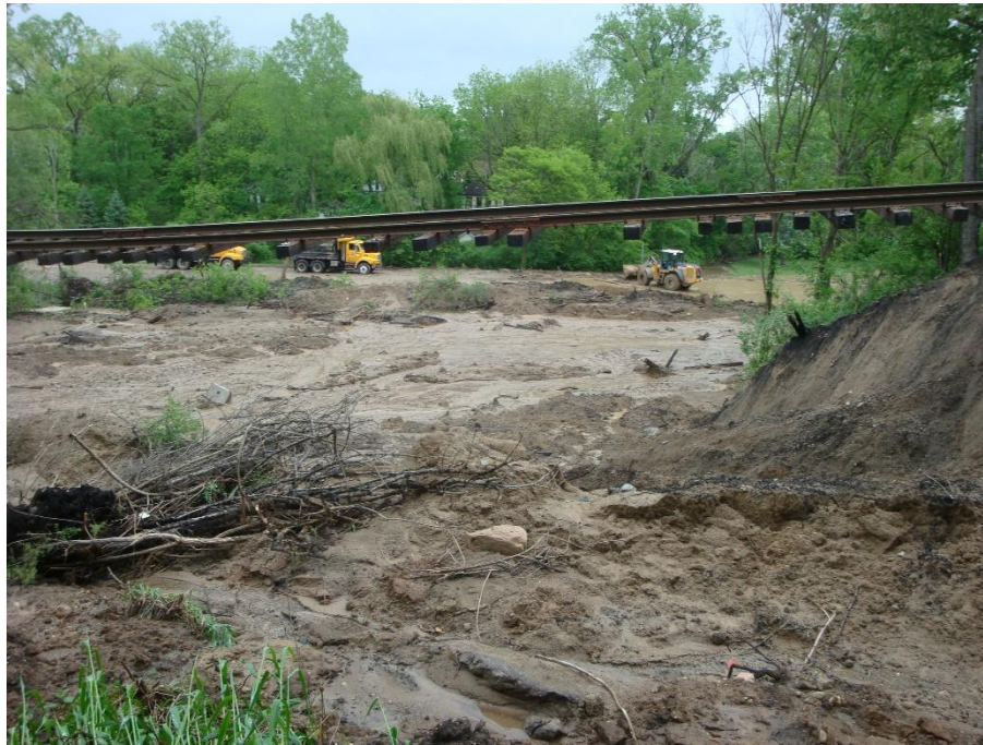
Figure 4. View of the conditions downhill of the failure showing deposition of debris and water. Trucks and dozer are operating on Plymouth Rd. and flooded area further back is a flooded public park.
