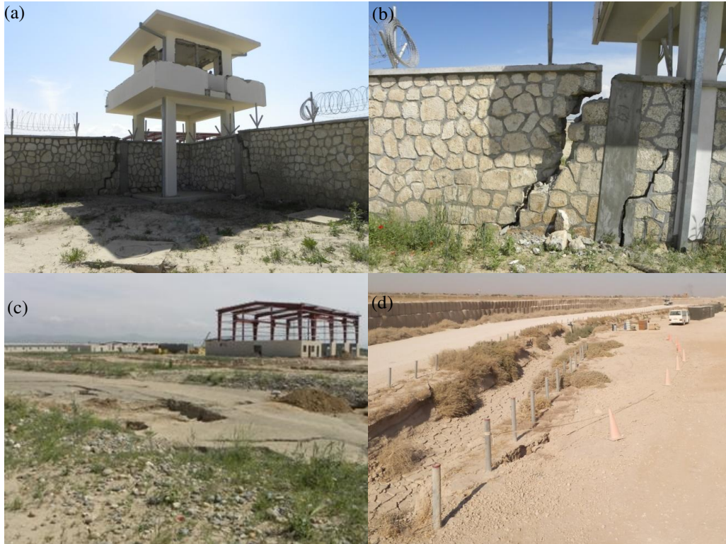
Figure 2. a. Damaged guardhouse and security wall in Kunduz, b. security wall damaged in Kunduz, c. settlement basin through a road in Kunduz, d. slope failure next to earthen drainage ditch in Mazar-e-Sharif as evidenced by coned off area.
