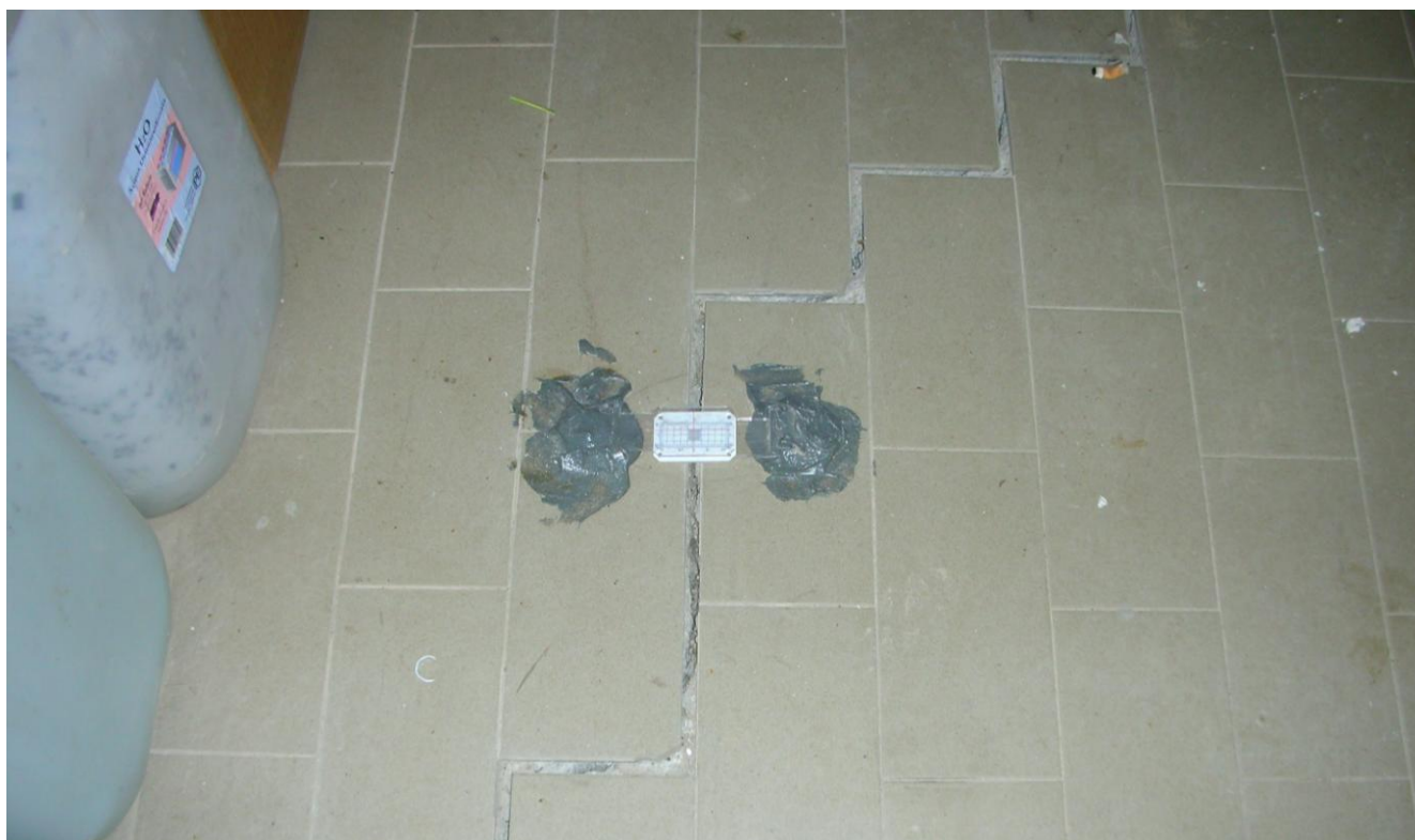
Figure 3. Floor damage inside the warehouse.
