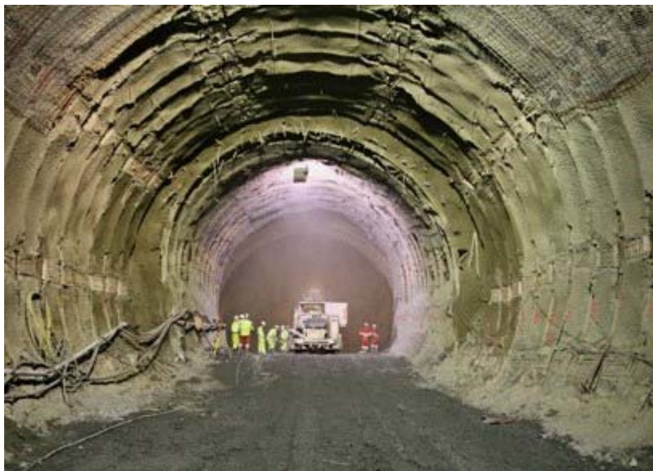
Figure 9. Photograph of the tunnel with the DSM support system installed. The HiDCon elements inserted in the shotcrete lining are well visible.
