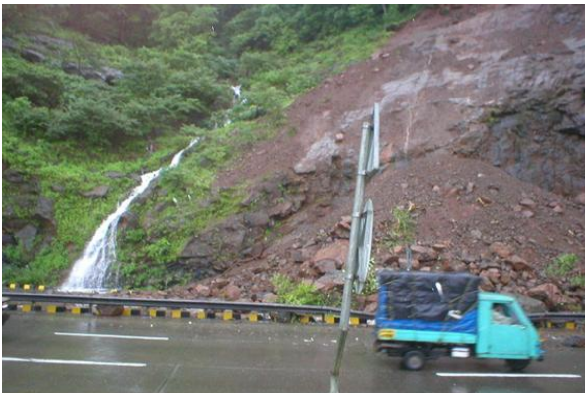
Figure 7. Significant water drainage during a monsoon.
