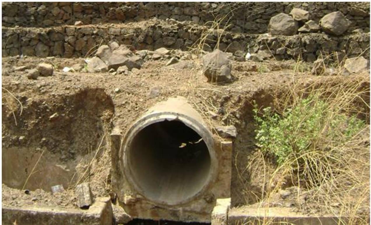
Figure 12. Pipe culvert without stepped chute.
