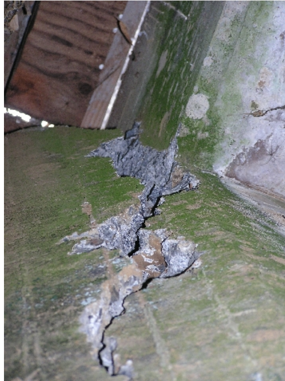
Figure 66. Location 20, bridge at approximately Mile Post 28, Hwy 270. At SW corner of bridge, looking upward at wooden plank sidewalk above. Fresh spalling of bridge abutment headwall at old, pre-existing cracks.
